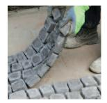
For a more realistic look you can interlock the Cobble Carpet Stones by cutting the half blocks. The Random Carpet Stones are also designed to be interlocked by simply cutting out the centre stone and turning the cut pieces 90° to join the mats together.
