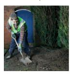
**STEP 2:** Cover the entire area with a semi-dry foundation mix of 6 parts sharp sand to 1 part cement. This should be 75mm deep. Compact and level the area. It is recommended that a maximum of 3m x 3m is levelled at any one time.
