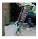
**STEP 3:** Lay the Carpet Stones as required, making sure the joints are evenly spaced. Use a rubber mallet to ensure the stones are well bedded into the foundation. Alternatively, you can use a 75mm x 50mm piece of timber with the rubber mallet. Use a spirit level to ensure the paving is level.
